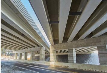
The project required extensive cooperation between County Materials, Lunda Construction, and WisDOT. Lunda Construction did the formwork and fabricated the templates, and County Materials tied the rebar cages and executed the pour. The team used one of County Materials' pouring beds to cast the pier elements.
