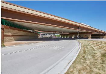
Project contractor, Lunda Construction was contracted to excavate the new road elevation, construct the Williamsburg Way bridge, and reopen the road in less than three months. The road was excavated 25 feet below, allowing traffic to pass under the soon to be constructed bridge. Originally, the contractor scheduled two days for the delivery of 22 prestress girders; however, incoming inclement weather conditions prompted crews to reschedule the delivery for a single day with one day's notice.
