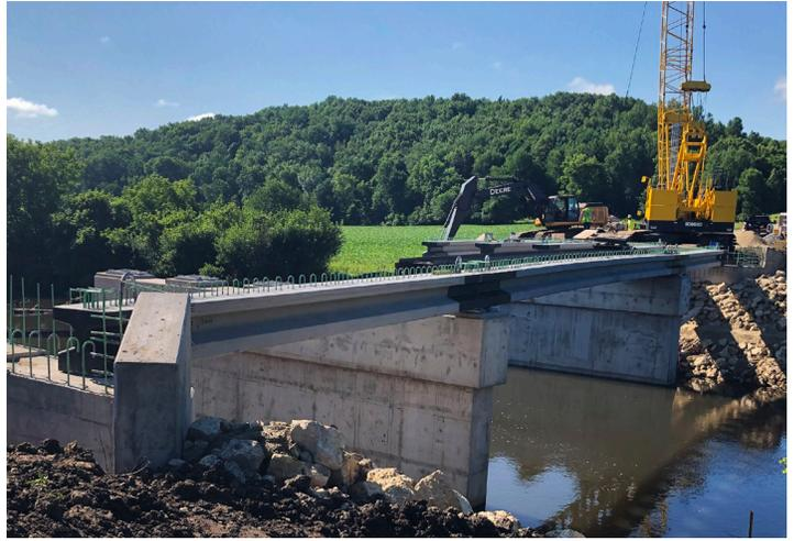
In addition to efficiency, prestressed bridge girders offer unmatched longevity. Their prestressed fabrication supports high load capacities through decades of inclement weather and heavy use. State departments of transportation rely on prestress girders for their extended service life, which can reach up to 100 years with minimal maintenance.
